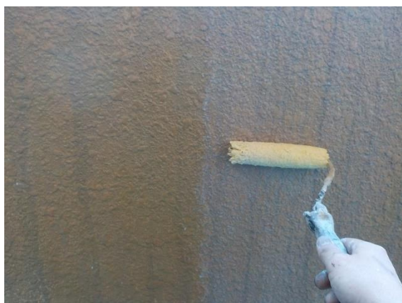
防水塗装壁面ﾌﾟﾗｲﾏｰ塗装状
